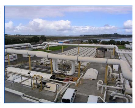
From 2001 to 2003 Maskell supplied buried process air pipework for the Project Manukau consortium, Manukau Wastewater Services, who have the Mangere WWTP upgrade project. Ductwork and piping for the \$360M project, in the DN450 – DN1500 range, was installed for process air piping. Further supporting information regarding Maskell capability and projects is available upon request.
